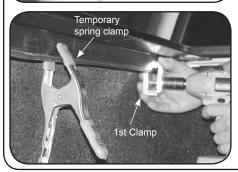
B. Hold rail in proper position with spring clamp. Install 1st clamp as close to front as possible and use 1/2" wrench to tighten.
