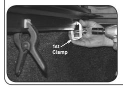
B. Hold rail in proper position with spring clamp. Install 1st clamp as close to front as possible and use ½" wrench to tighten.
